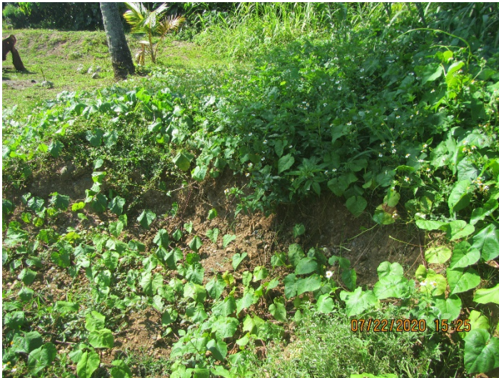
Photograph 3: IMG_1344: This photograph is a close-up of the berm indicated by the red arrow in Photograph 2: The vegetation in the forefront of this photo appears to be Pueraria Montana as identified in the USACE Site Visit Report (Appendix D). Pueraria Montana is a facultative species.
